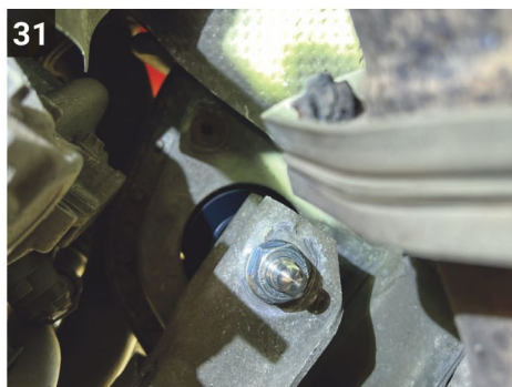
31 If the engine dropped slightly when you unfastened the old mount, simply raise it a few millimetres to ensure you have enough bolt thread to work with.
